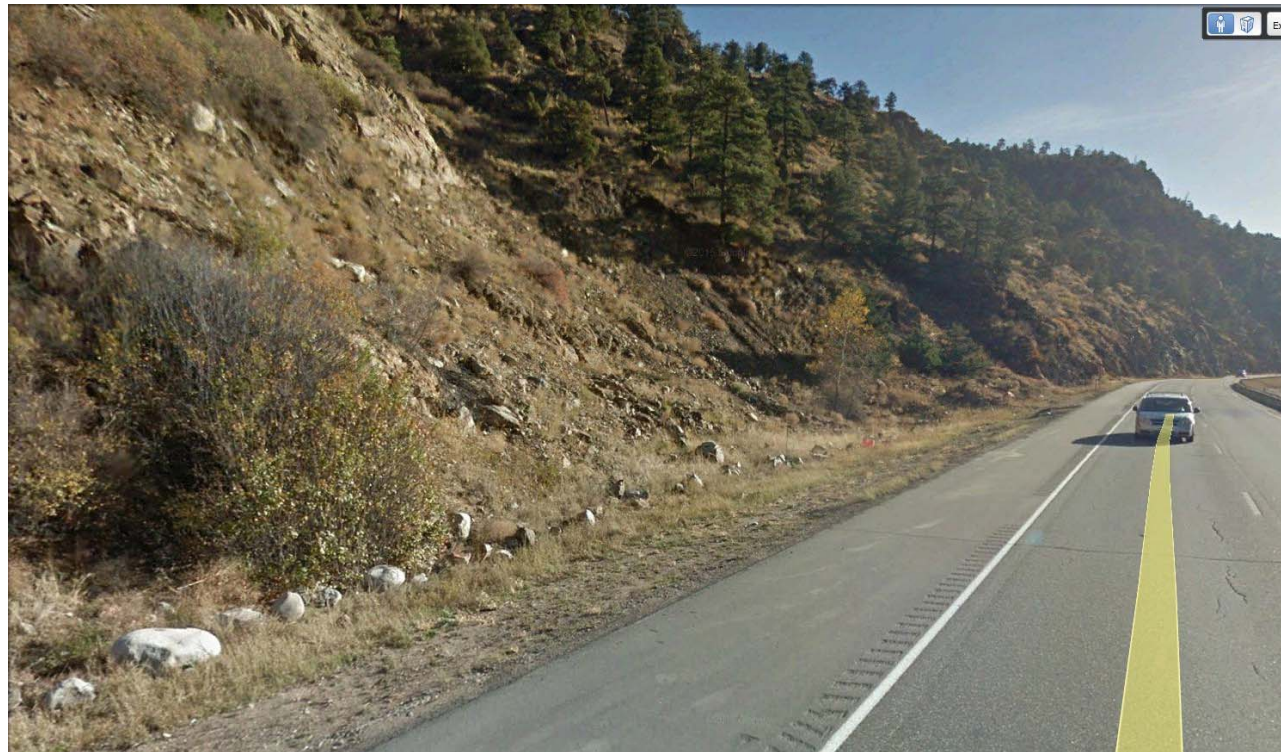
EXAMPLE: EXISTING ROCK CATCH DITCH JUST EAST OF DUMONT
