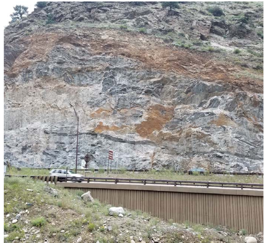
EXAMPLE: ROCK CUT WITH MESH EAST OF THE VETERAN'S MEMORIAL TUNNELS
